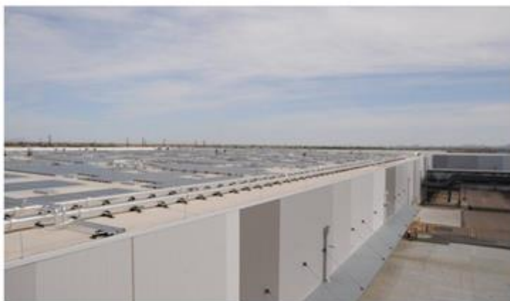
Apple's new command center in Mesa, AZ, should help fuel demand for new data centers in the Phoenix region for years.
